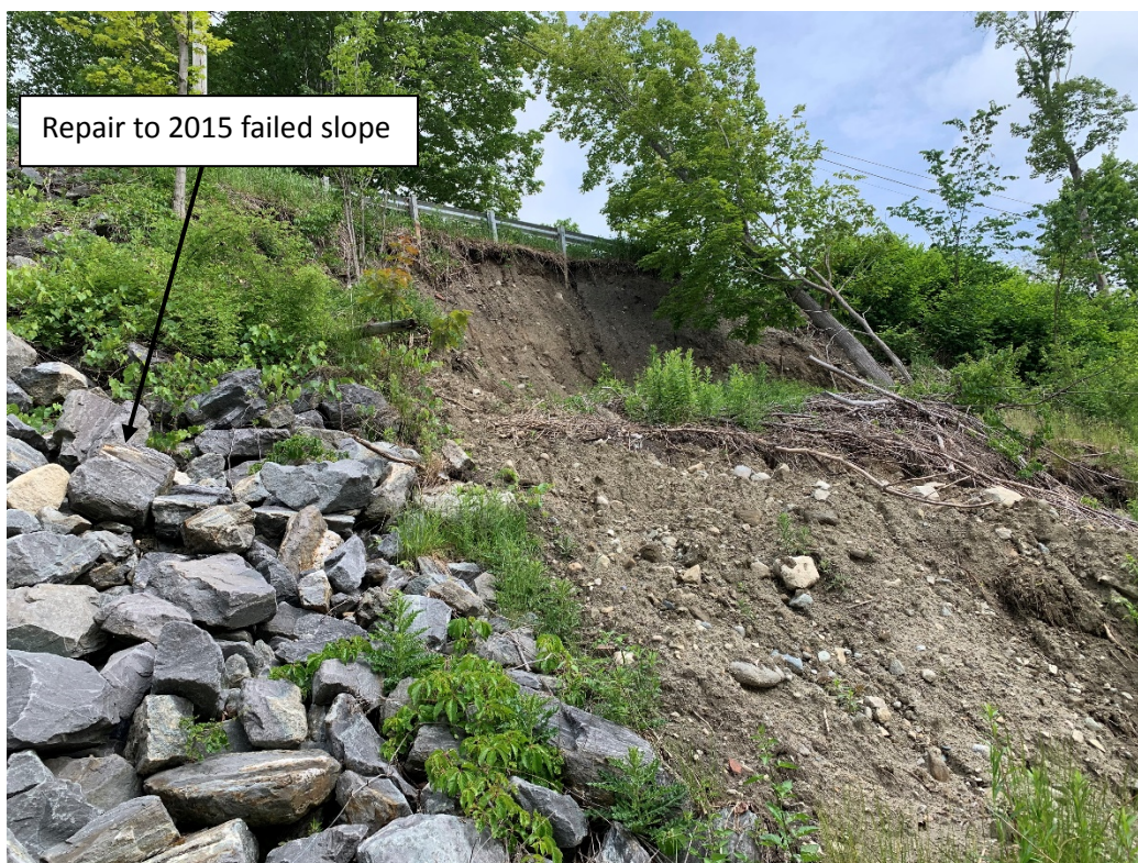
Photo 2 – Top section of failed slope on June 8, 2023
