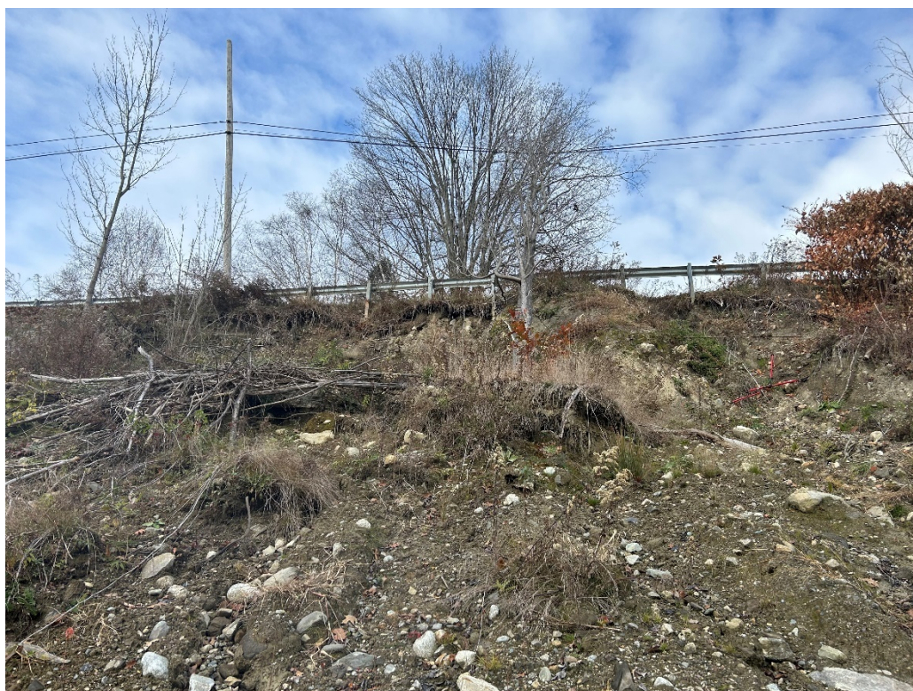
Photo 8 – Sloughed embankment soils on November 14, 2023
