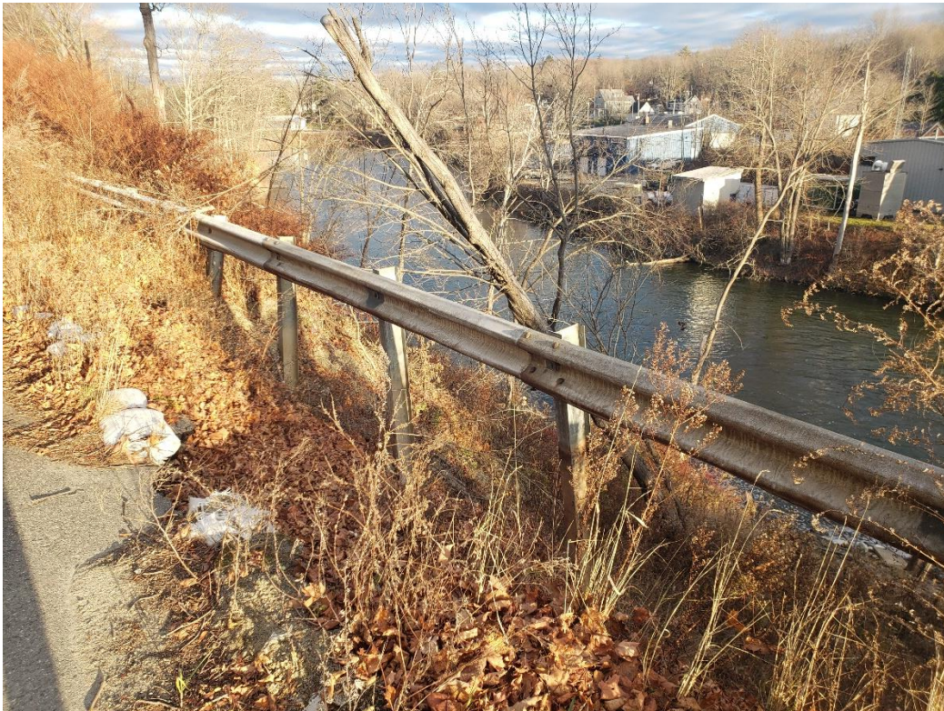
Photo 8: Guardrail and road edge at top of slope failure. Looking east.
