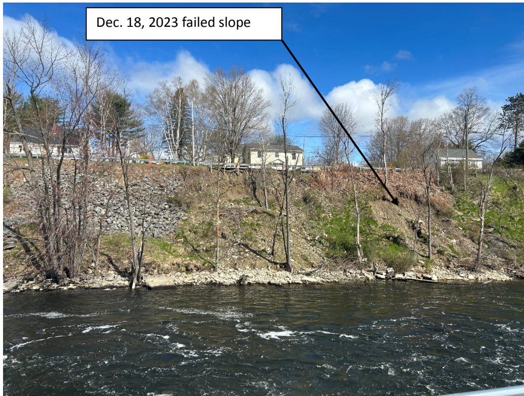
Photo 3 – Failed Slope on May 3, 2024.
