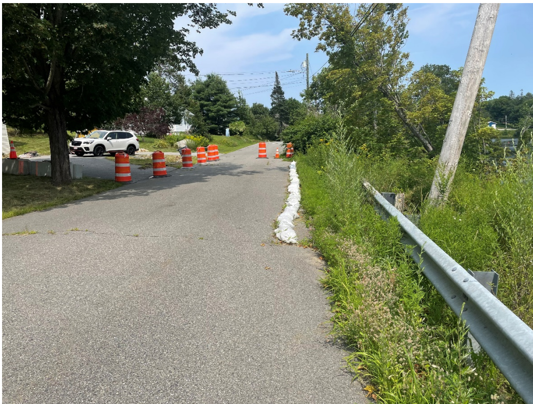
Photo 7 – Rotated utility pole and tree on overhead utility lines of August 3, 2023
