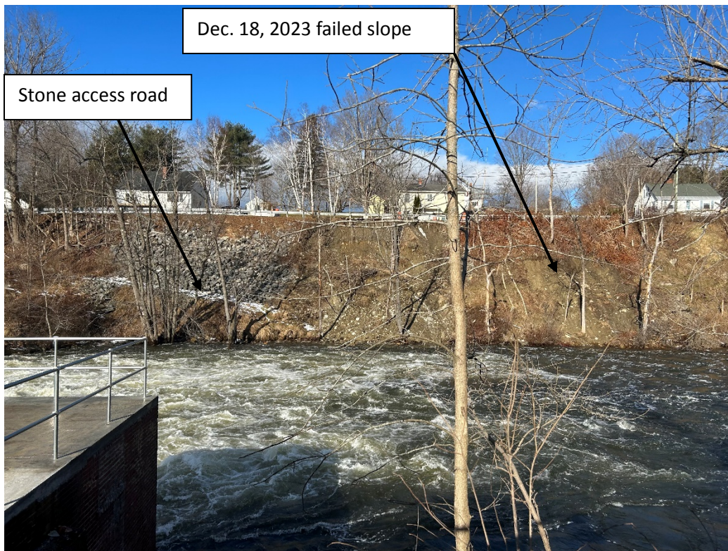
Photo 2 – Failed slope and stone access road on January 12, 2024
