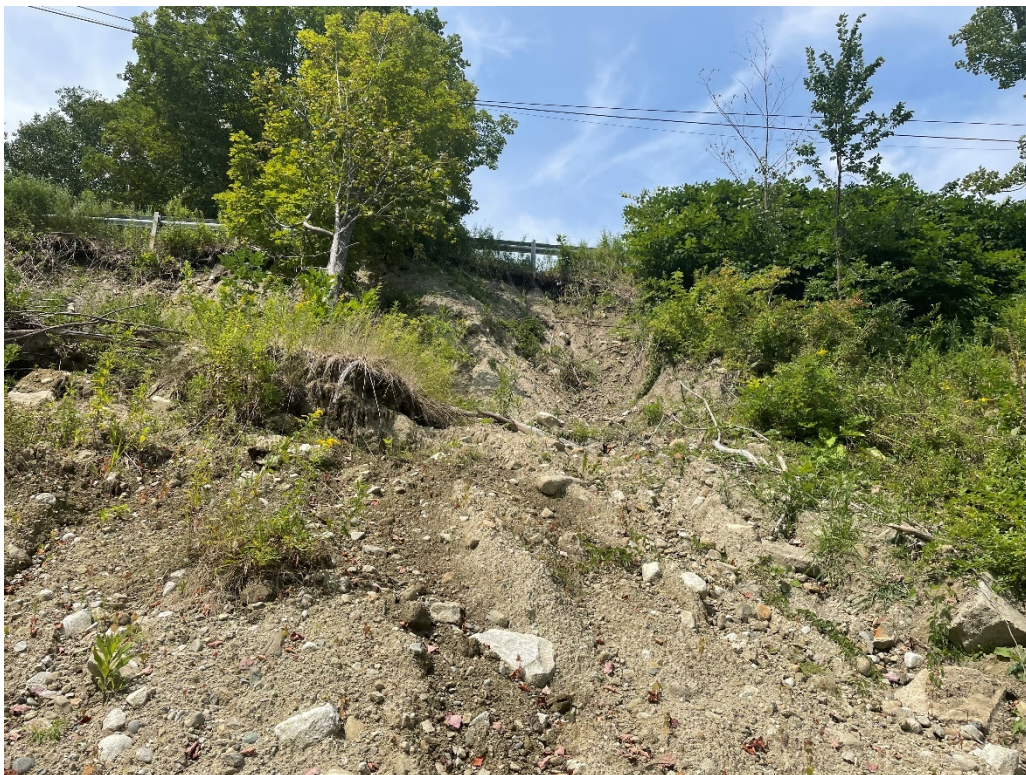
Photo 6 – Sloughed embankment soils on August 3, 2023
