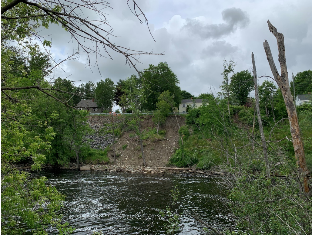
Photo 3 – Failed Slope from east side of Cobbosseecontee Stream on June 8, 2023.
