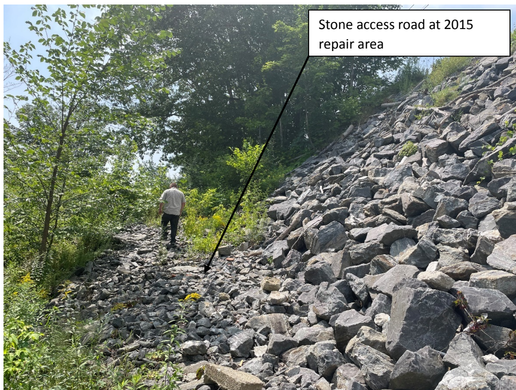
Photo 4 – Section of slope repaired after 2015 failure on August 3, 2023
