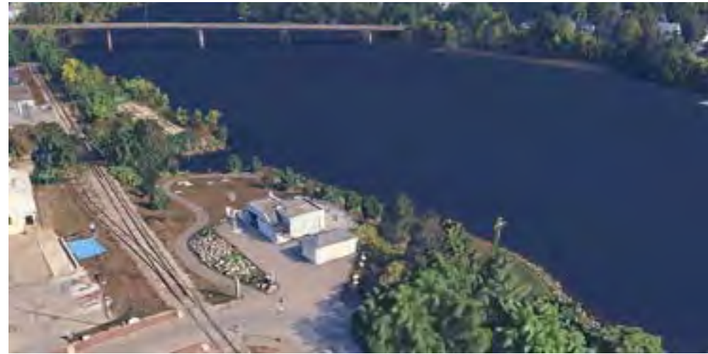
B | Maine Ave Pump Station
