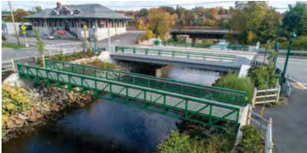
D | Pedestrian Footbridge
