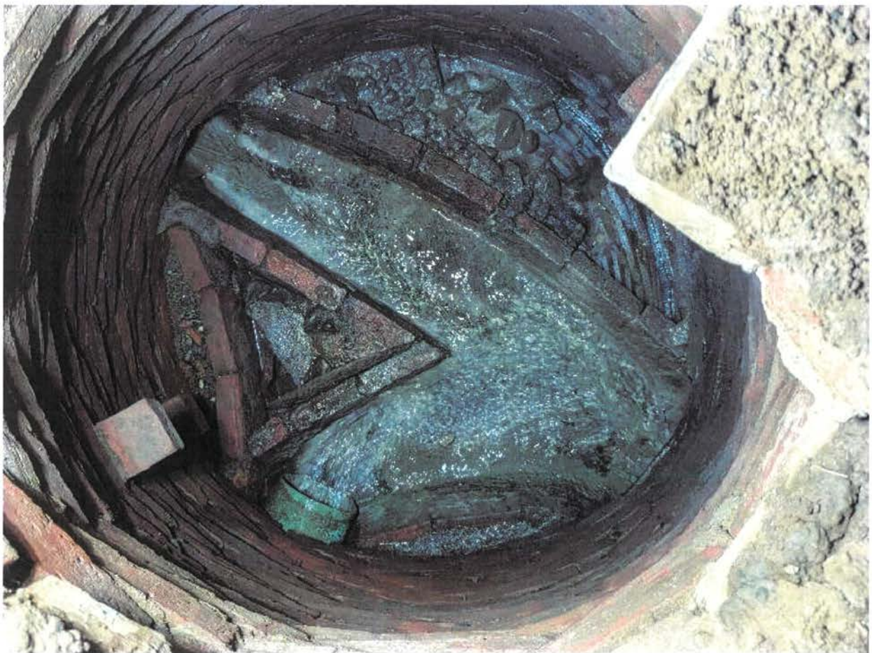
Winter Street Sewer
