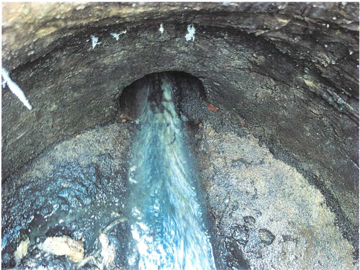
Harrison Avenue Sewer
