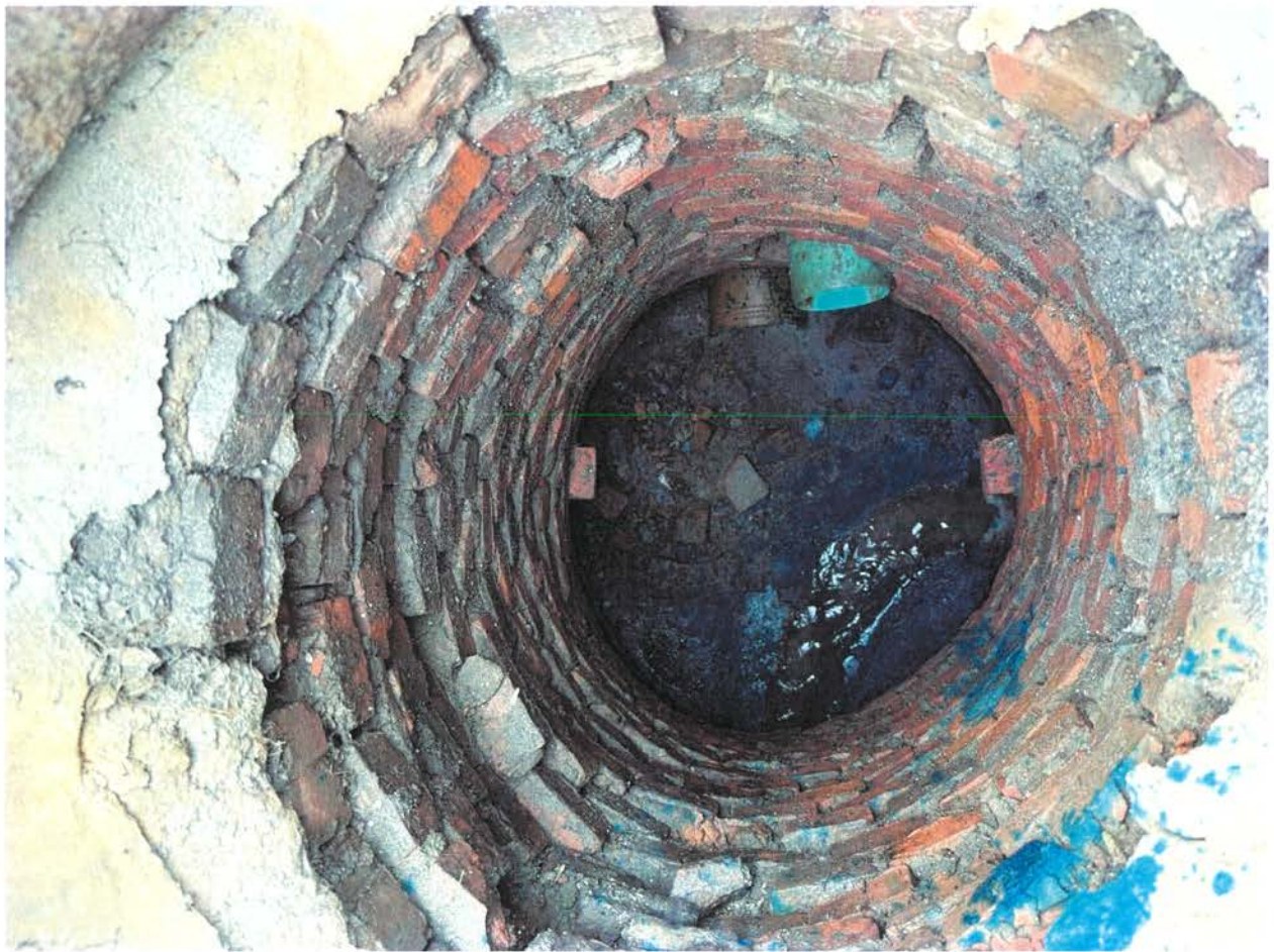
Kingsbury Sewer at River Avenue
