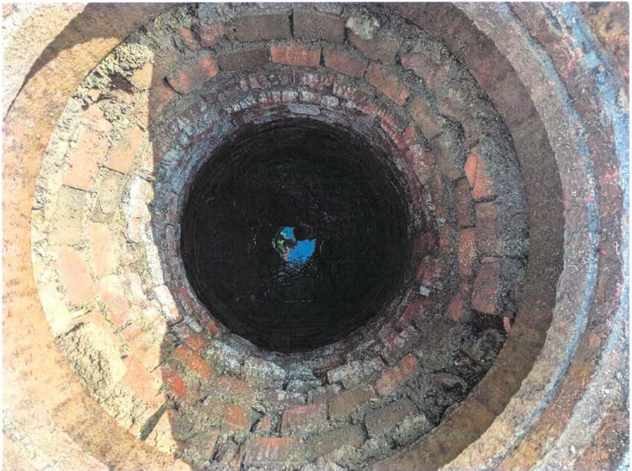
Cannard Street Sewer
