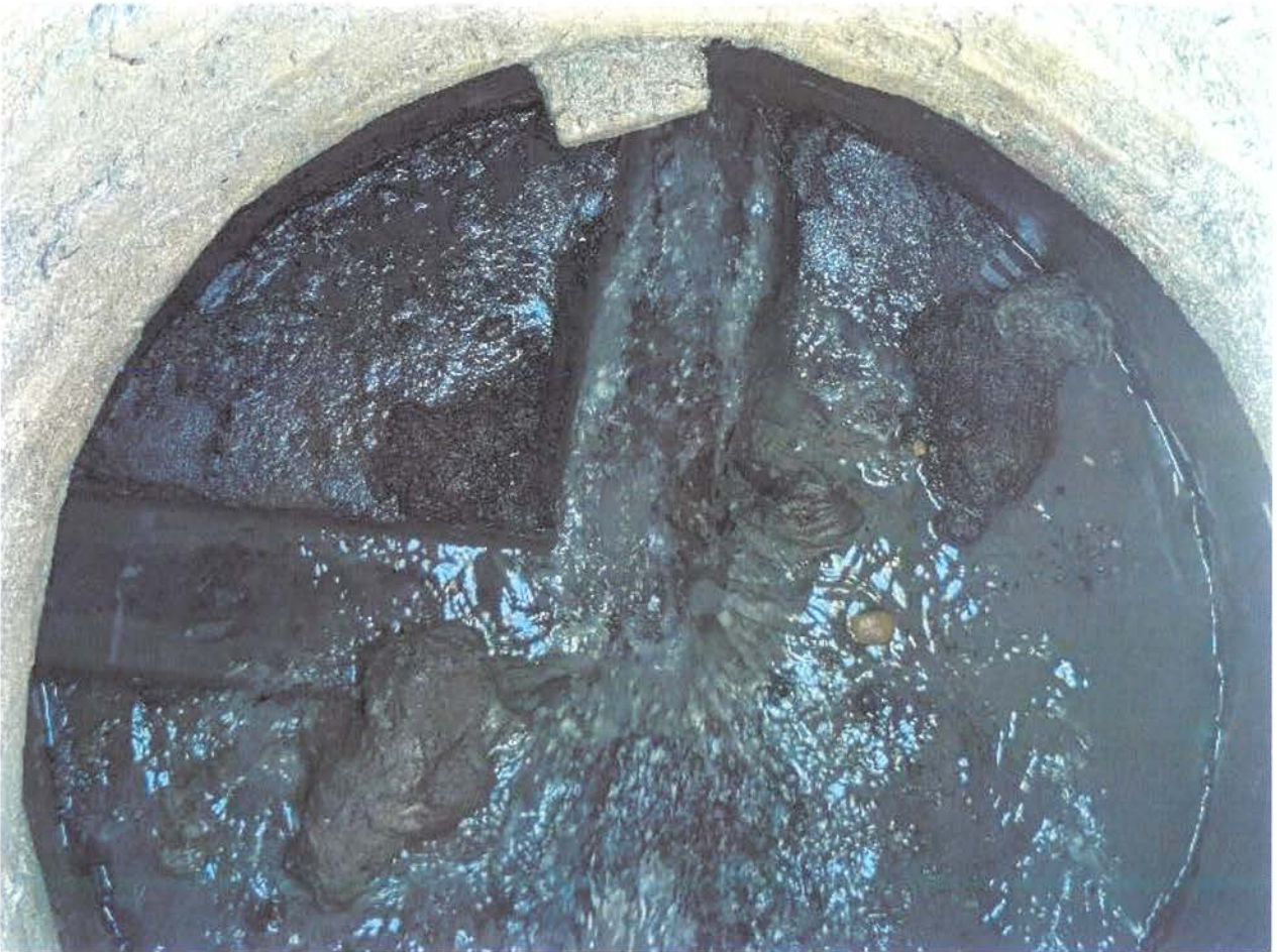
School Street Sewer
