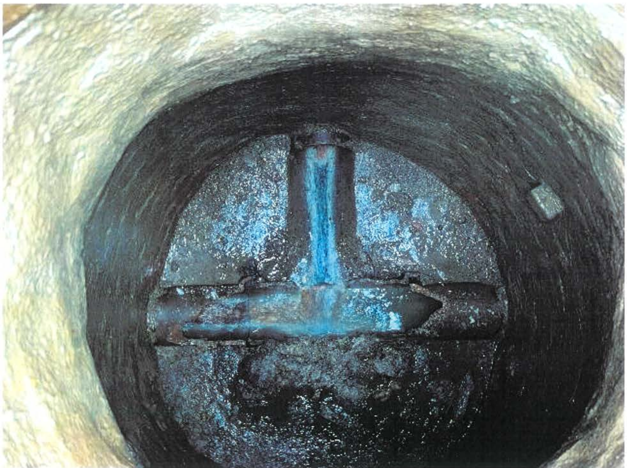
Plaisted Street Cross-Country Sewer
