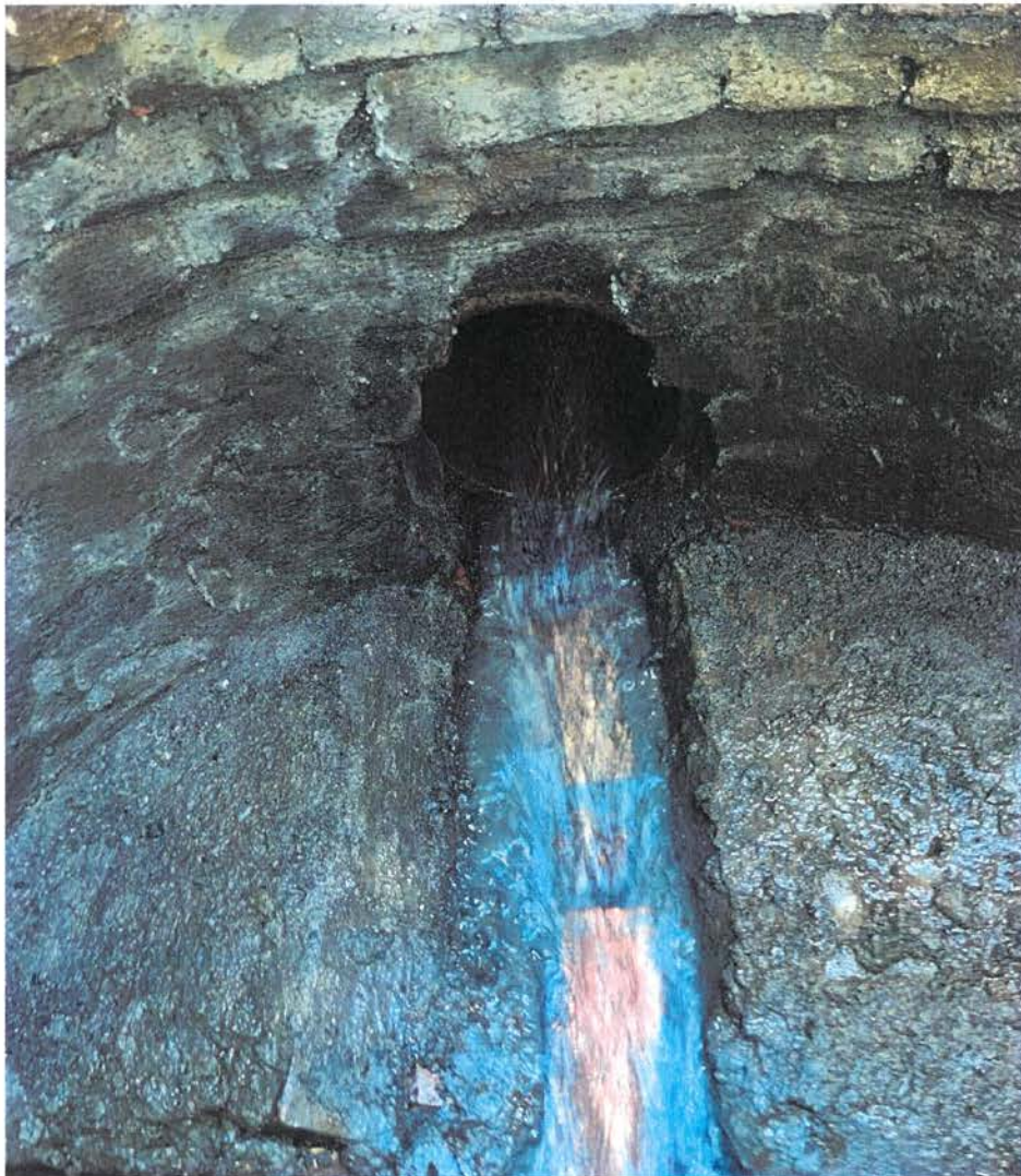
Central Street Sewer
