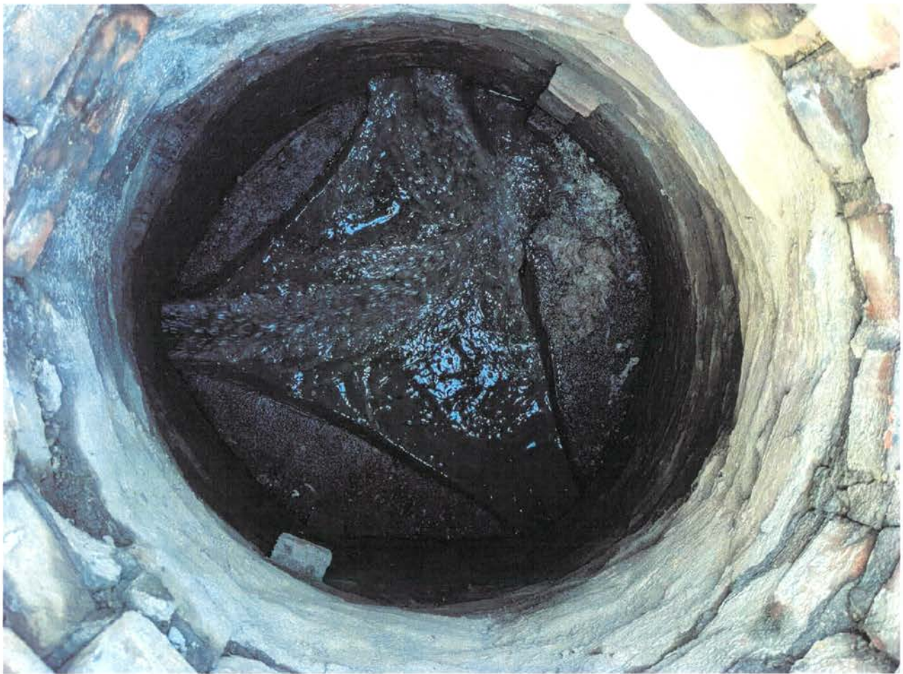
Lincoln Avenue Sewer
