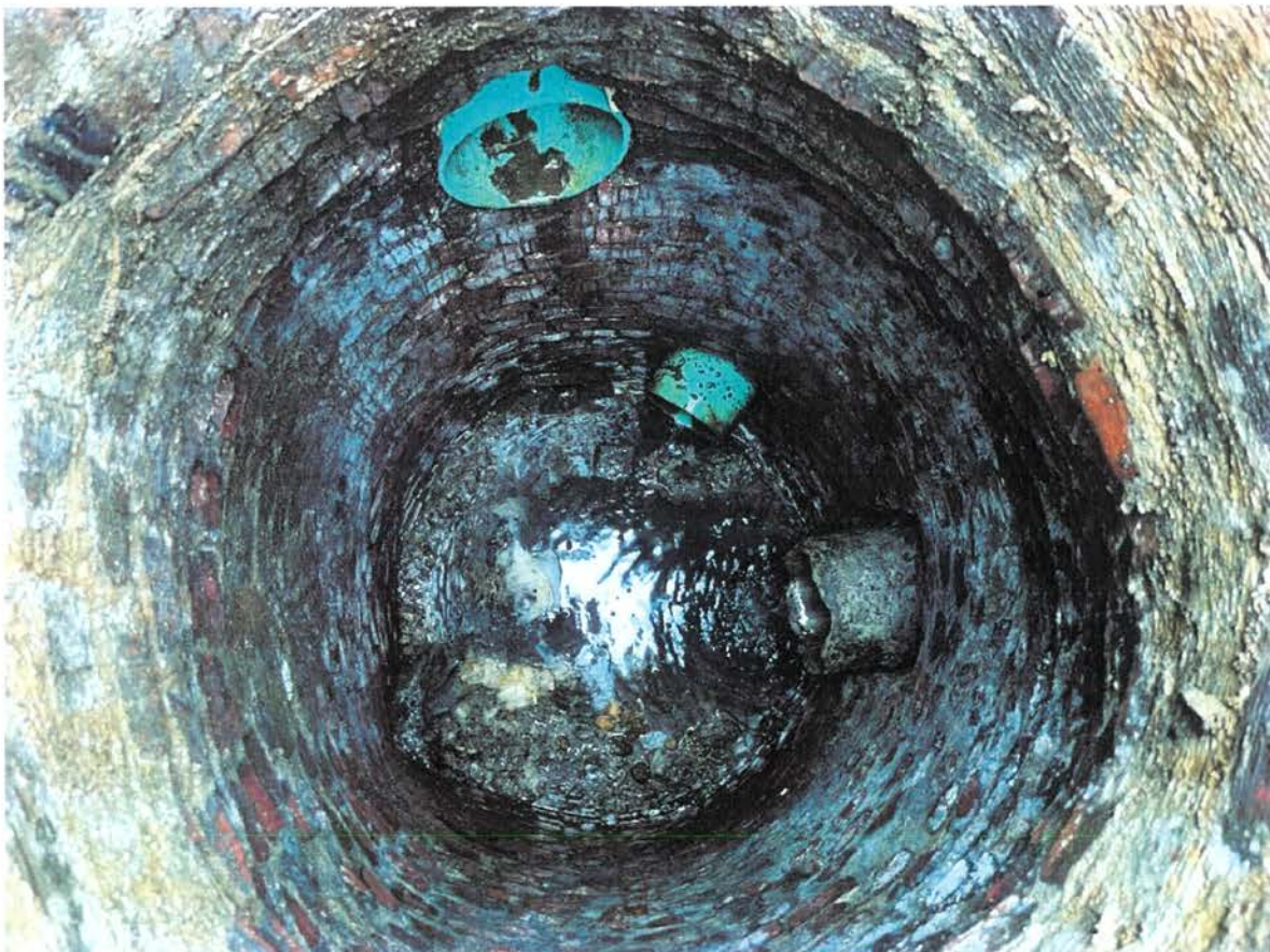
Spring Street Sewer
