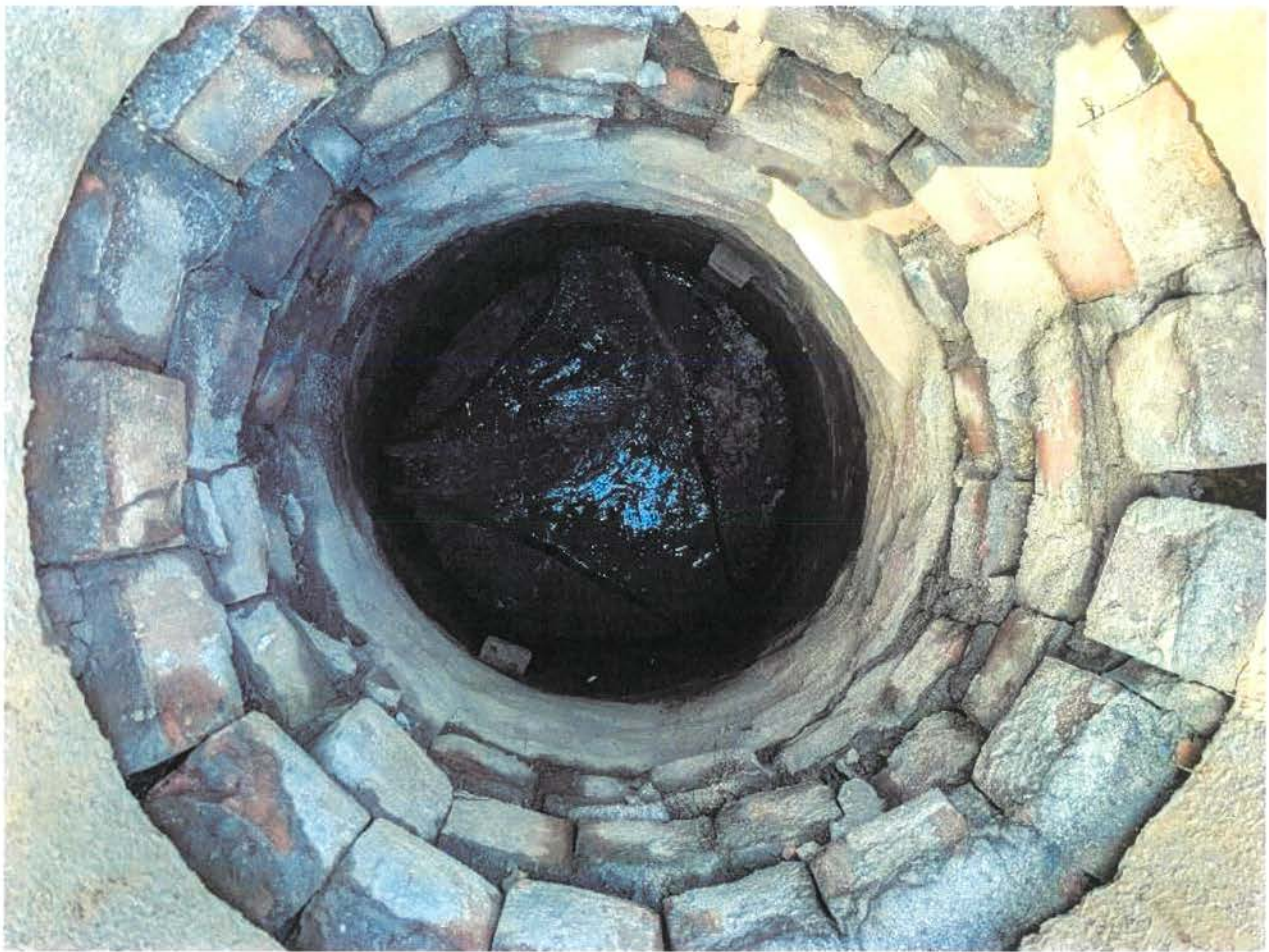
Fremont Street Sewer
