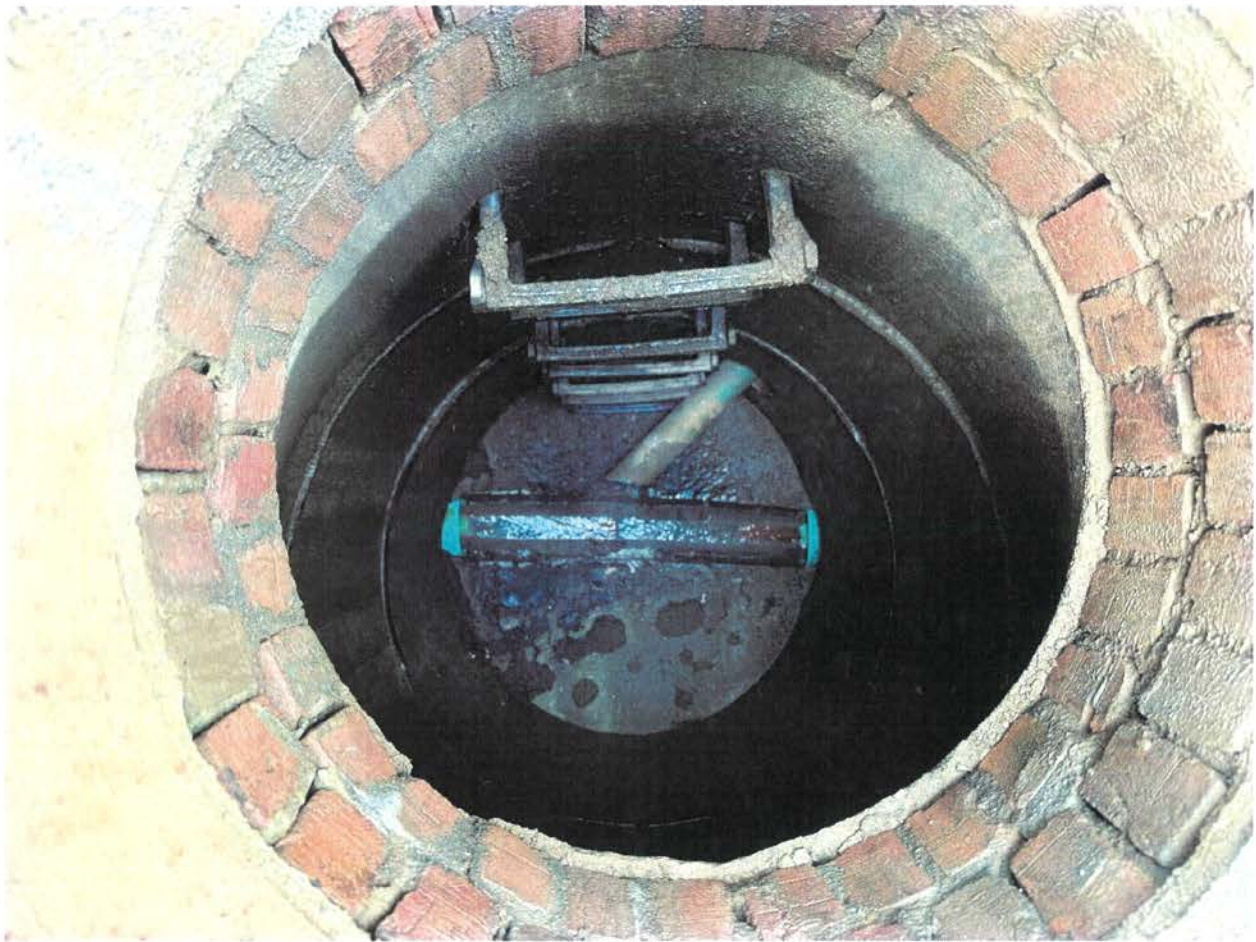
Bowman Street Sewer
