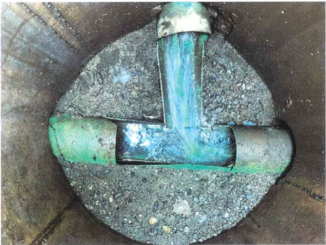
Harden Street Sewer
