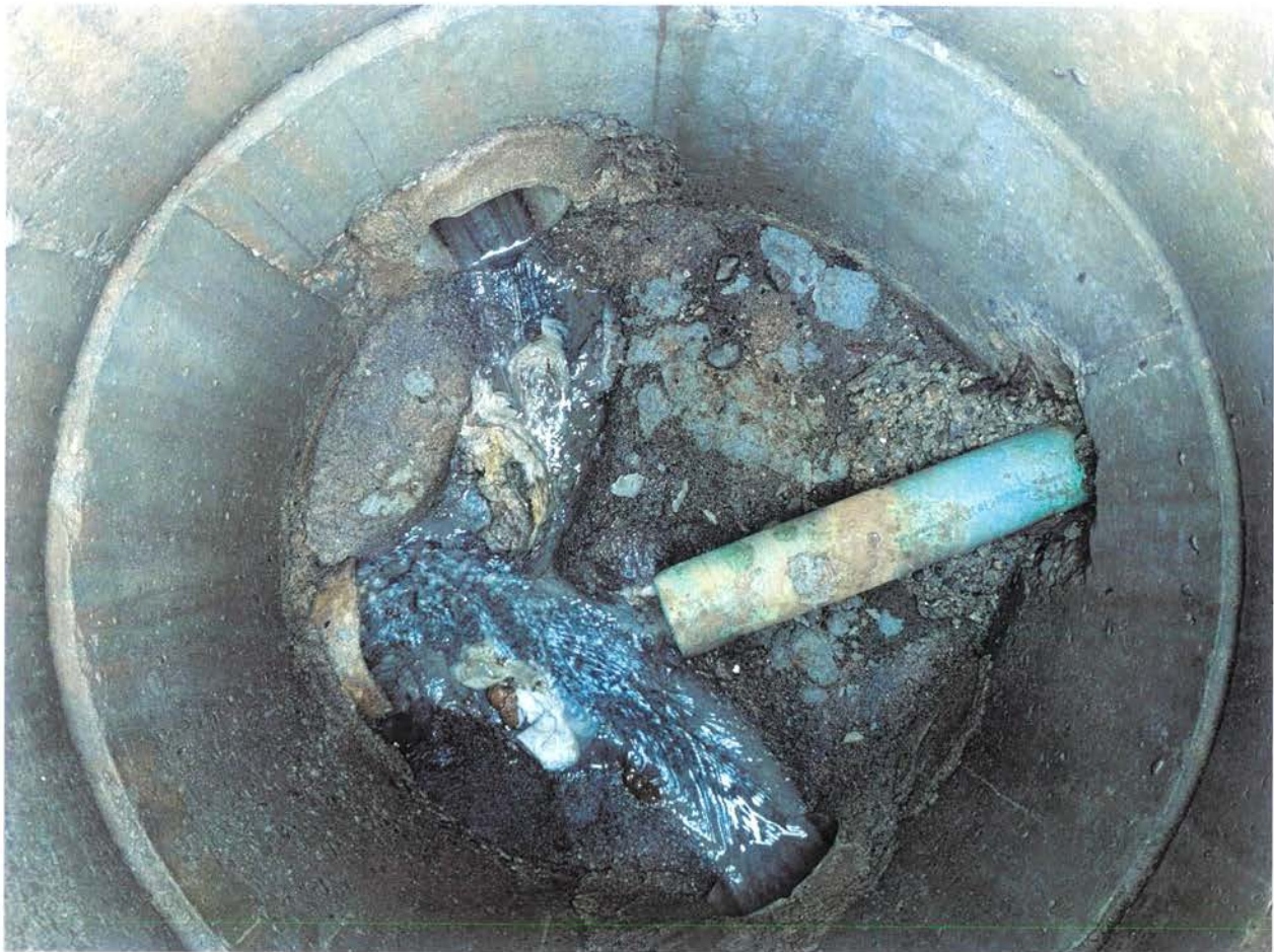
Ash Street Sewer
