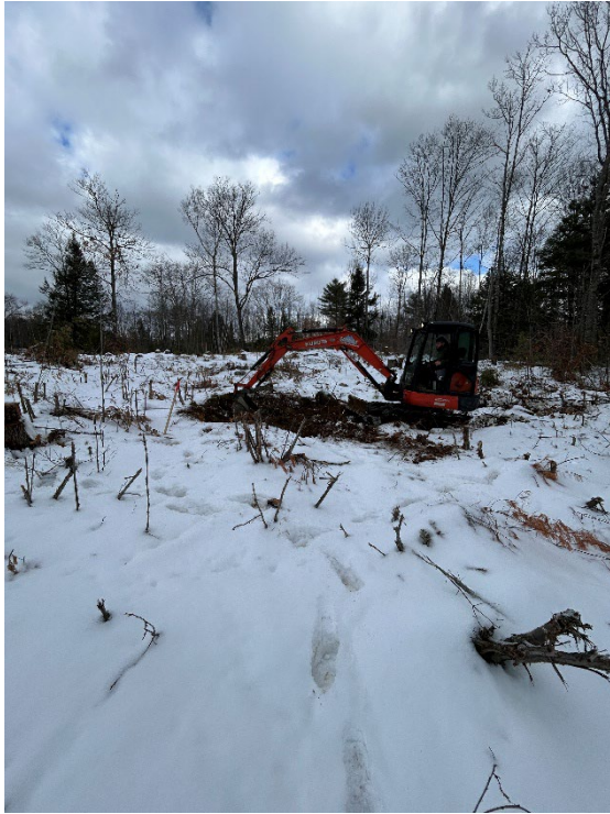
Test Pit TP- 8 Facing North
